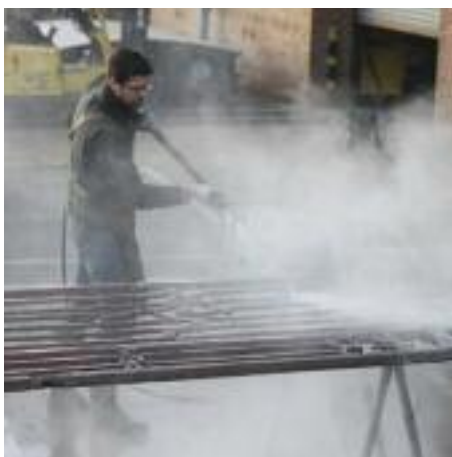
Initial cleaning of gates
